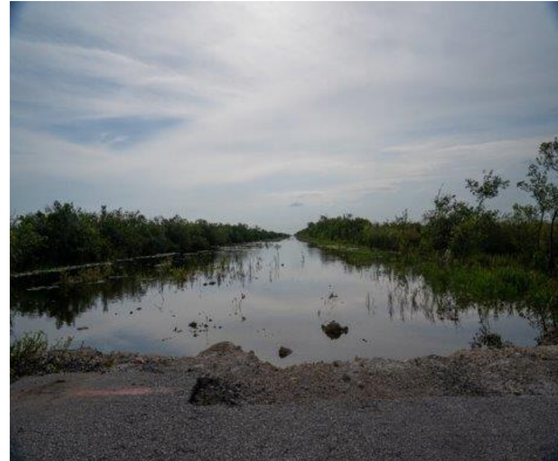
Old Tamiami Trail Roadbed Removal
