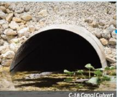
C-18 Canal Culvert
