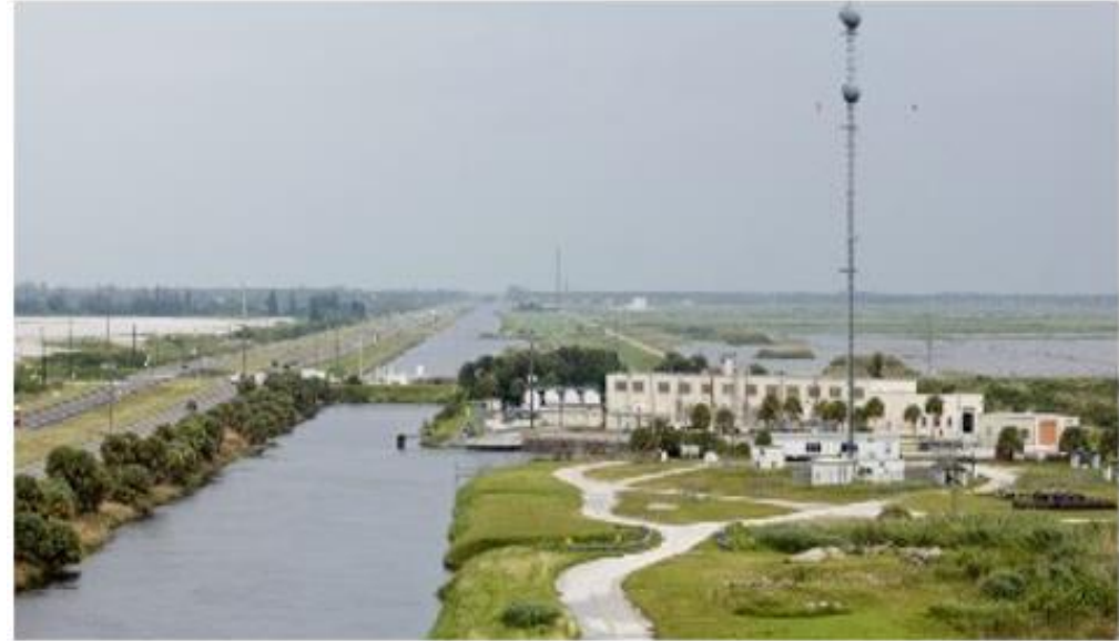
Modern Day S-5A Pump Station
